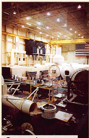
Construction de la station ALPHA.
